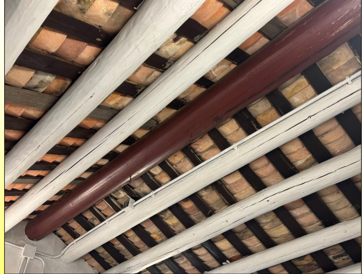
木椽和桁條 Timber rafters and purlins
