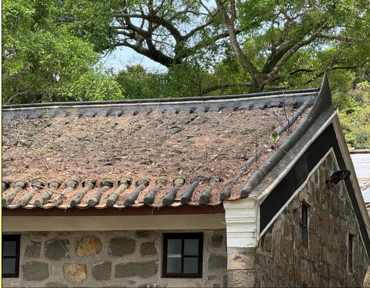
鋪砌了客家瓦的傳統硬山頂 Traditional flush gable roof laid with Hakka-style tiles
